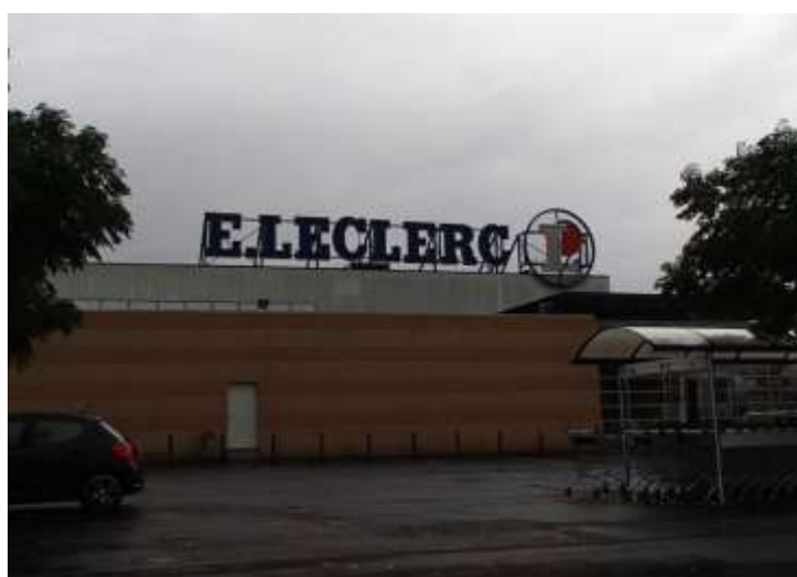
Structure insuffisamment dissimulée
